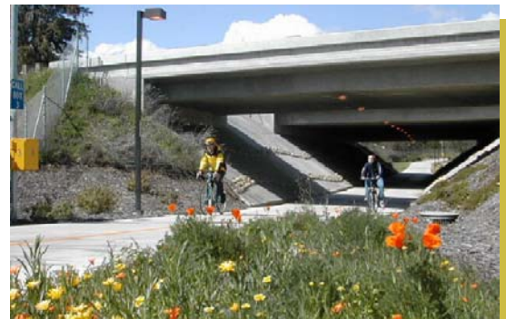
Type 4 Grade-Separated Undercrossing
