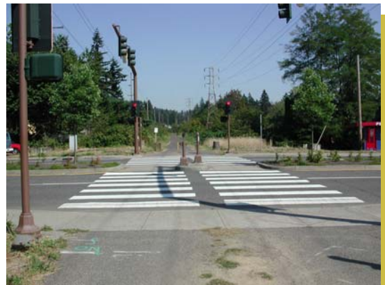
Signalized crossing at 82 nd Ave and 122 nd Ave in Portland (OR) includes: two marked crosswalks (one for each movement); landscaped median with signal activation; pedestrian and equestrian push button activation; bicyclist loop detector signal activation; good sight lines; and advance warning signs for motorists.
