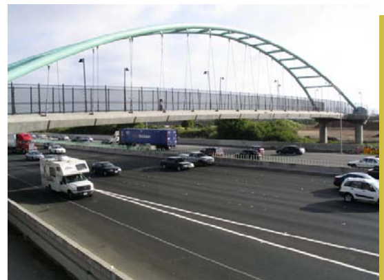
Type 4 Grade-Separated Overcrossing
