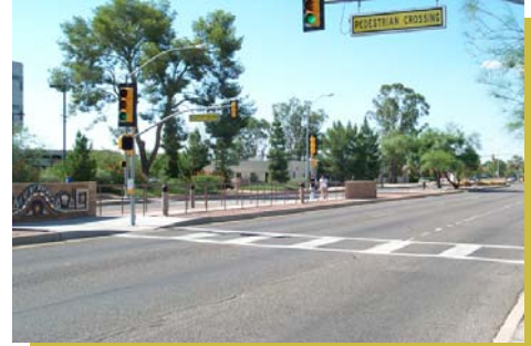
Pelican signal in Tucson, AZ
